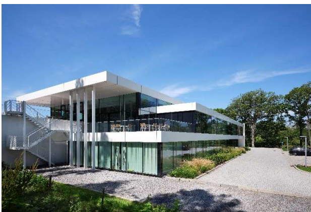
Headquarters of LASEA in Liège (Belgium)
